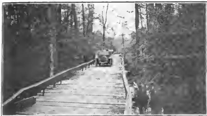
Pathfinder Crossing a Bridge Near Corinth, Mass.
